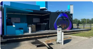
Installing technology and cabling elements
