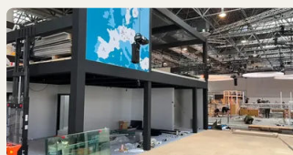
Fit-out: glazing and large display
