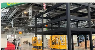
Column grid and deck beams
