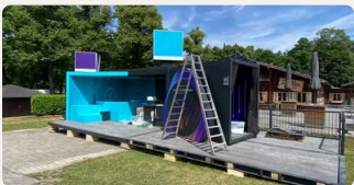
Building the deck and the top-mounted elements
