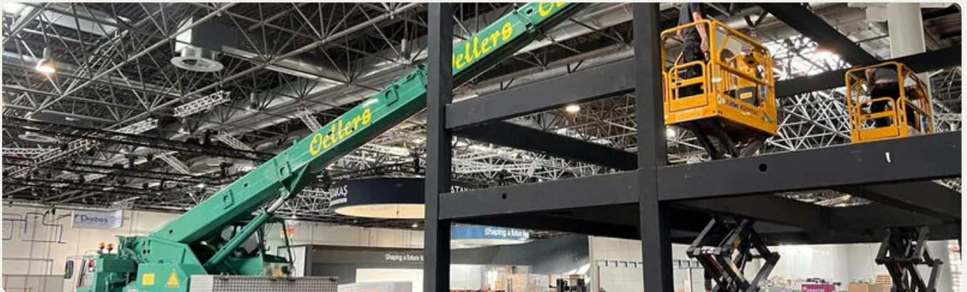
Assembly in the hall: build-up exactly to project documentation
