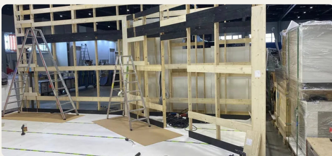
SHELL Timber frames erected, two levels
